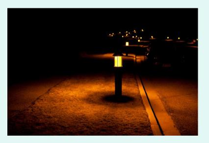
Much of the street lighting in Tekapo uses full cut-off bollards with low pressure sodium lamps. These are ideal for minimizing light pollution.
